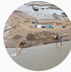
Dredging and Land Reclamation
